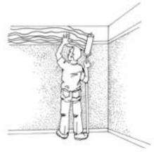
Starting from the centre, use a suitable tool to press the wall covering into the adhesive to expel all the air. Make sure that the tool you choose for smoothing out the wall covering does not damage it
