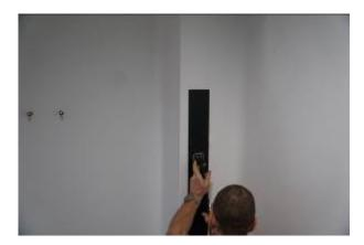
Apply adhesive right up to the horizontal line. See sections 1 and 4 and the adhesive manufacturer's instructions for application, use and drying times.
